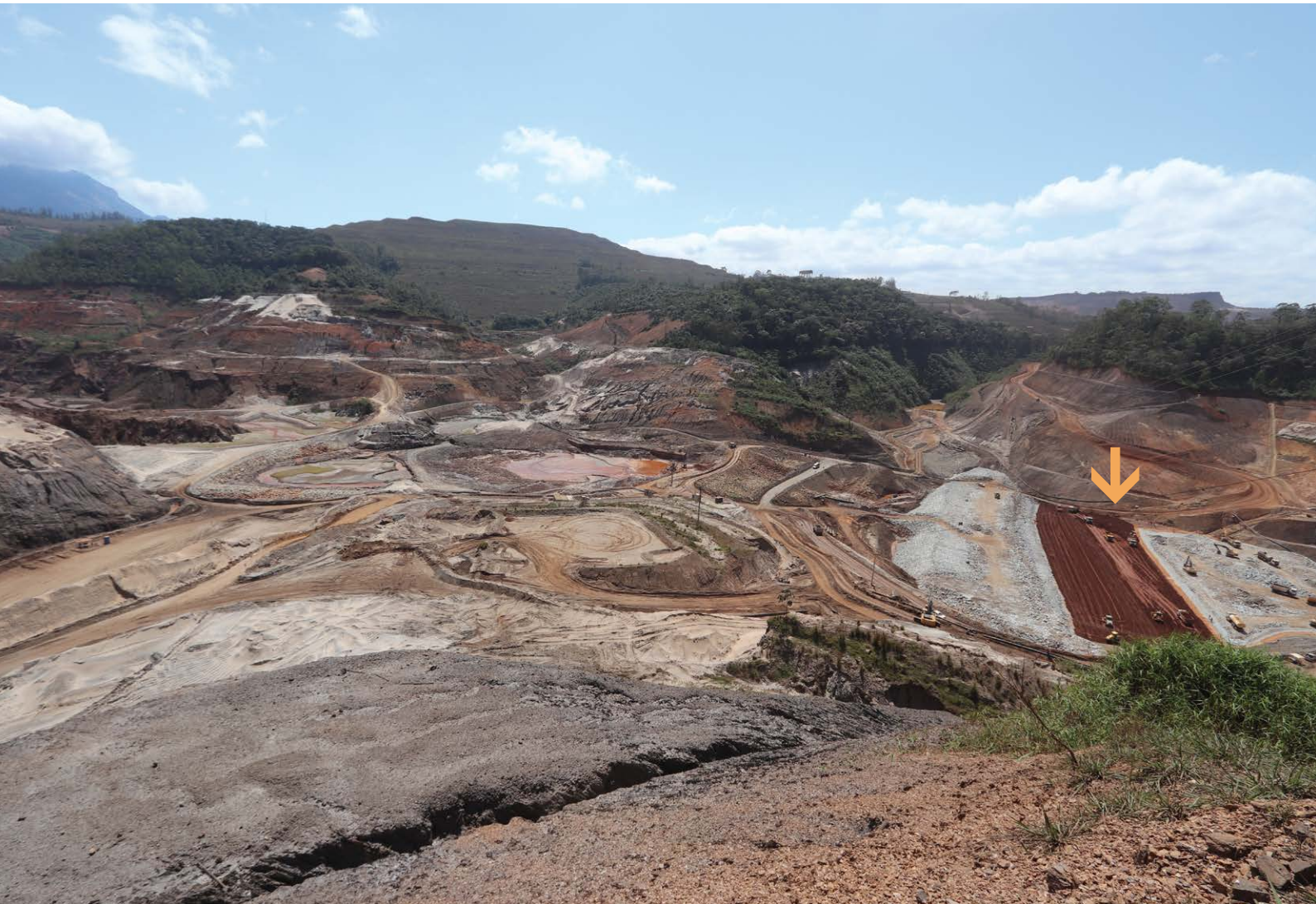
Figure 1. View of Fundão Dam site. On the right, a permanent dam referred to as S1, is being constructed to contain the tailings remaining on site. This dam is part of the actions determined by government agencies to address tailings management (October 2018).
